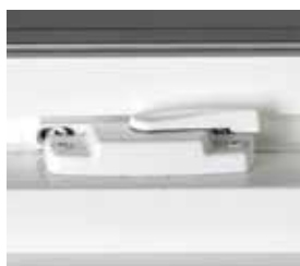
Cam Lock and Keeper
